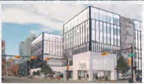
Joffre Place 6-story renovated office-to-residential conversion featuring 119 modern rental units
