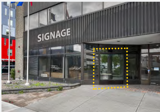
Future entrance for Unit 2
