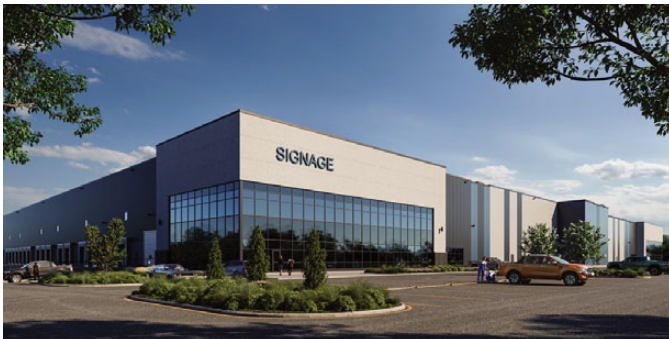
Metro Logistics leased approximately 291,000 square feet in Citylink Logistics Centre (60 Carmek Drive SE)
