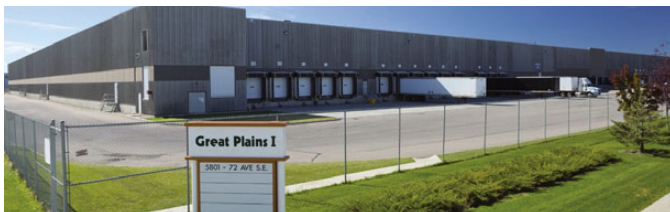
Continental Tire leased 70,000 square foot in Great Plains Industrial Park – Building 1.
