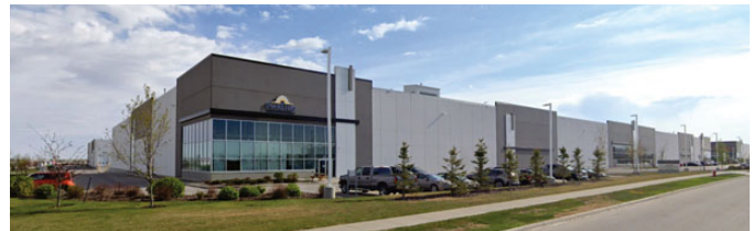
Fastlane Logistics leased 117,000 square foot in Nose Creek Business Park – Bldg. C.
