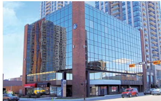
Stephenson Building on 11th Avenue SW – Beltline troublemaker
